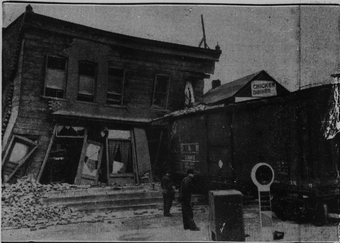
A freight car jumped the track and crashed into this restaurant on Jefferson Street, Schenectady, N. Y. Here is the scene after the crash, which all but demolished the building, and which sent two men to the hospital with serious injuries. (Central Press)
