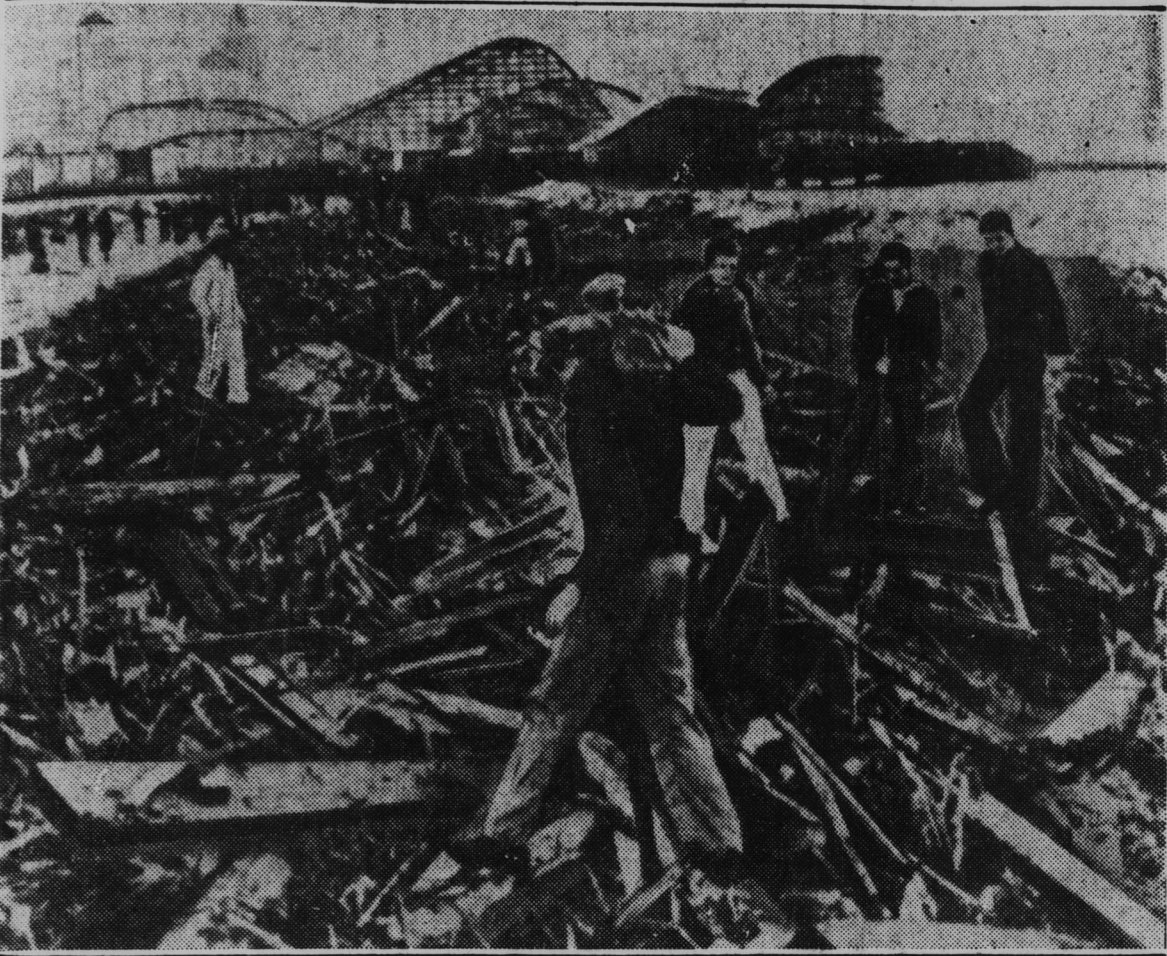
The beach near the mouth of the Los Angeles River at Long Beach is shown above, littered with tons of lumber and wreckage floated down by the raging waters of the disastrous flood. Thousands of valley residents are homeless—their homes piled on the beach by the flood waters.
