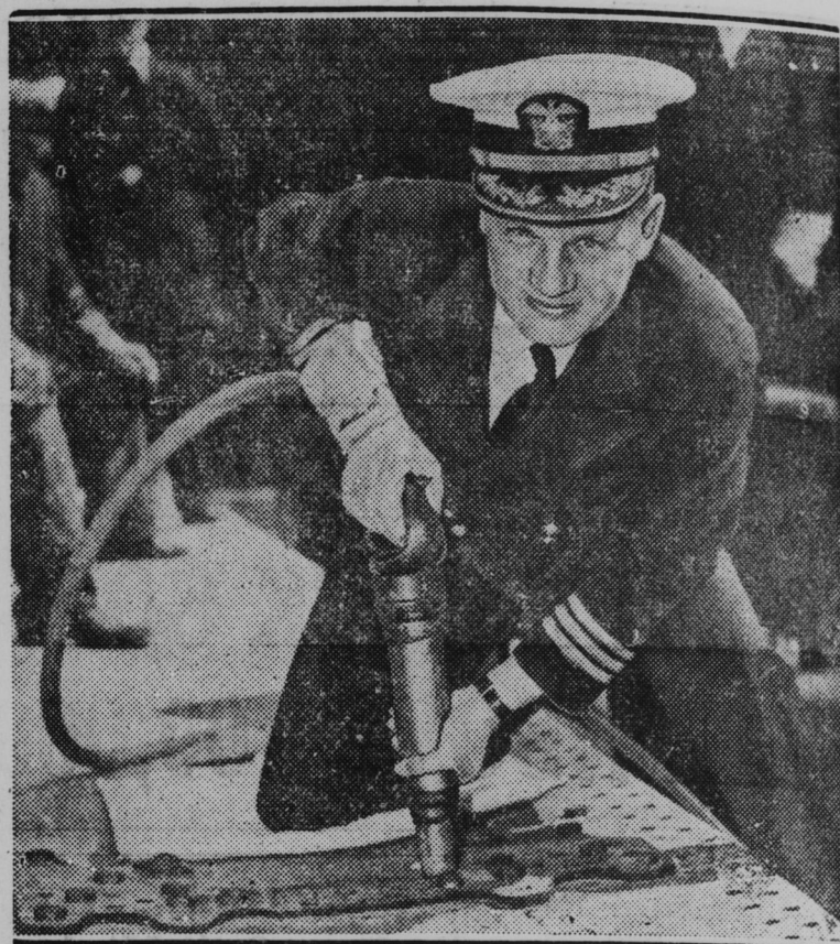
Using a riveting hammer to drive the first bolt, Commander Claude O. Kell, of the Charlestown, Mass., navy yard, is pictured beginning construction of the new U. S. destroyer Walke. Two destroyers are being built there. (Central Press)
