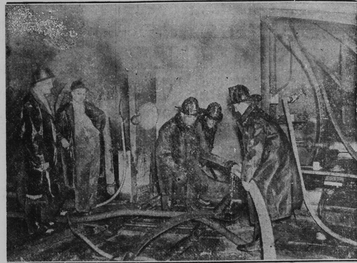
Braving suffocation and drowning, firemen are shown dragging lines of hose into the section of the midtown Queens vehicular tunnel where a fire raged. For a time the collapse of the entire $58,000,000 project was feared, but the blaze was eventually subdued by careful flooding of the tunnel. Compressed air was pumped in to keep the walls from breaking down.
