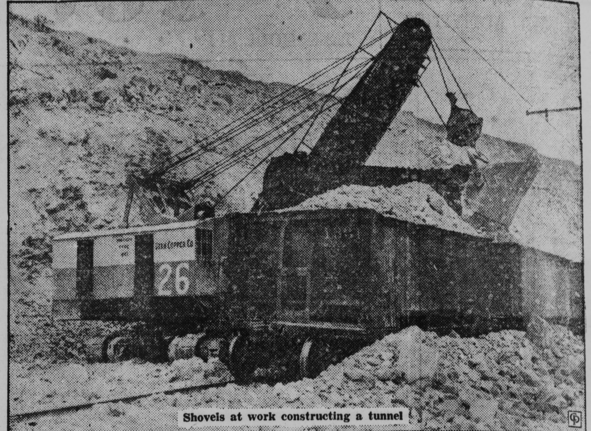
Shovels at work constructing a tunnel
