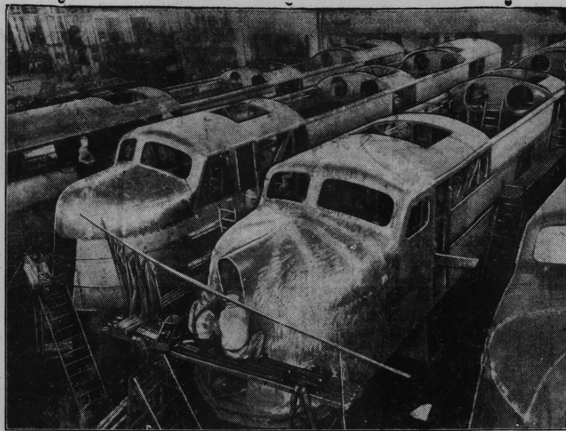
NEW SEABOARD RAILWAY FLEET TAKES FORM—Construction of the nine new 1800 horsepower Diesel-electric locomotives of the Seaboard Railway is progressing rapidly at the plant of the Electro-Motive Corporation, LaGrange, Ill.
