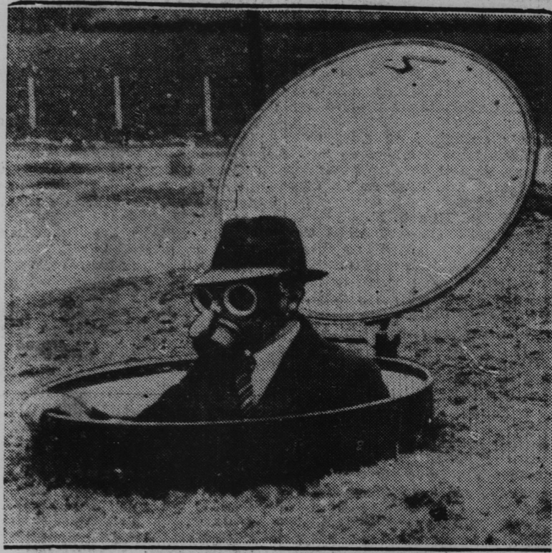
Hundreds of underground shelters have been constructed in the London area to take care of a large portion of the city's population in case of gas or air raids. A Londoner, wearing gas mask, descends into the chamber by way of a vent opening on a city park.
