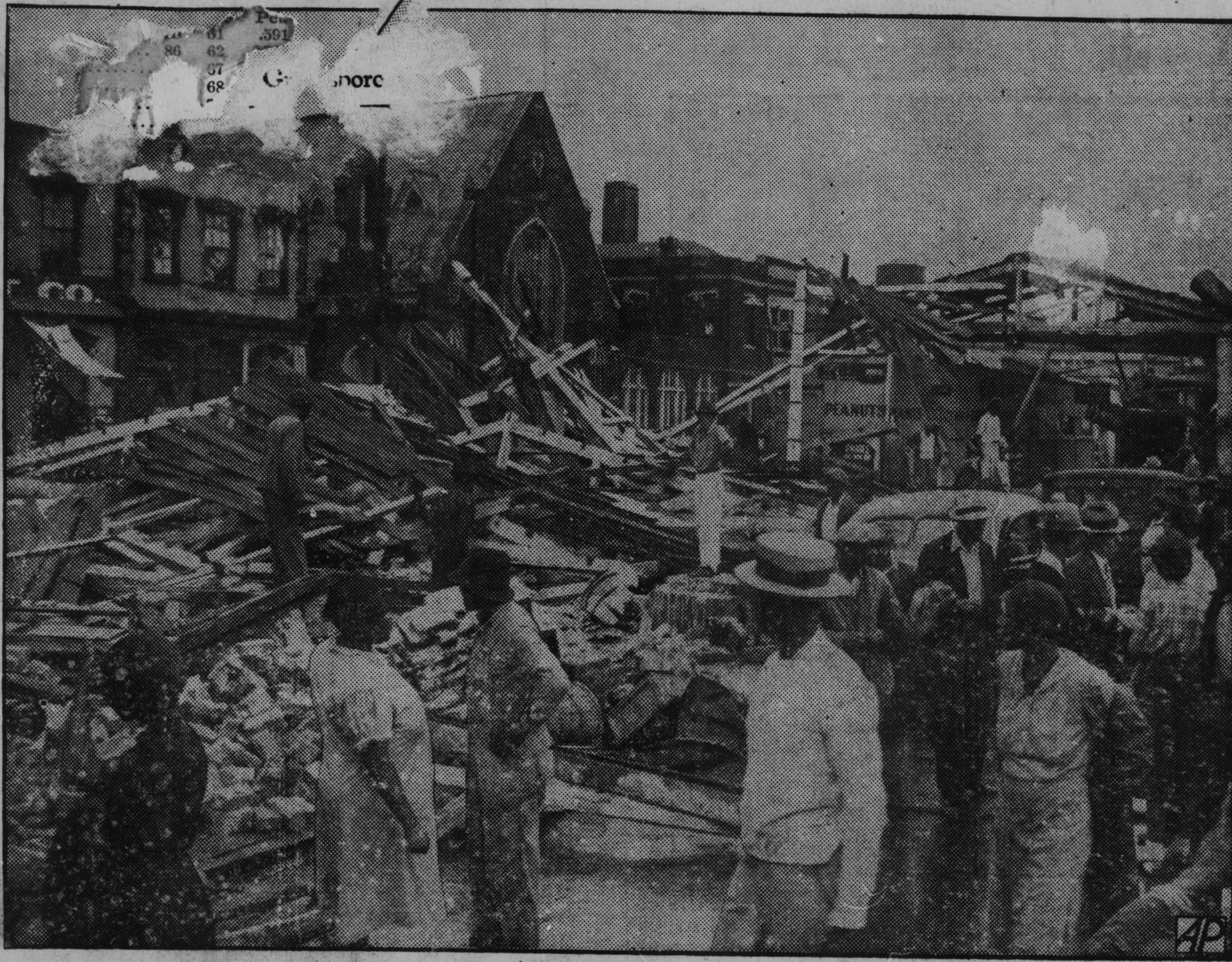
Swooping savagely on historic Charleston, S. C., a tornado killed 28 persons, injured 200 others and razed many buildings, including the City Market, for years a landmark. Several perished and many were hurt when the long building, extending from the business section to the waterfront, was reduced to a shambles. This picture shows wreckage at the east end of the market. The undamaged building and the adjoining chapel shown at the left constitute the Harriott Pickney Home for Seamen.
