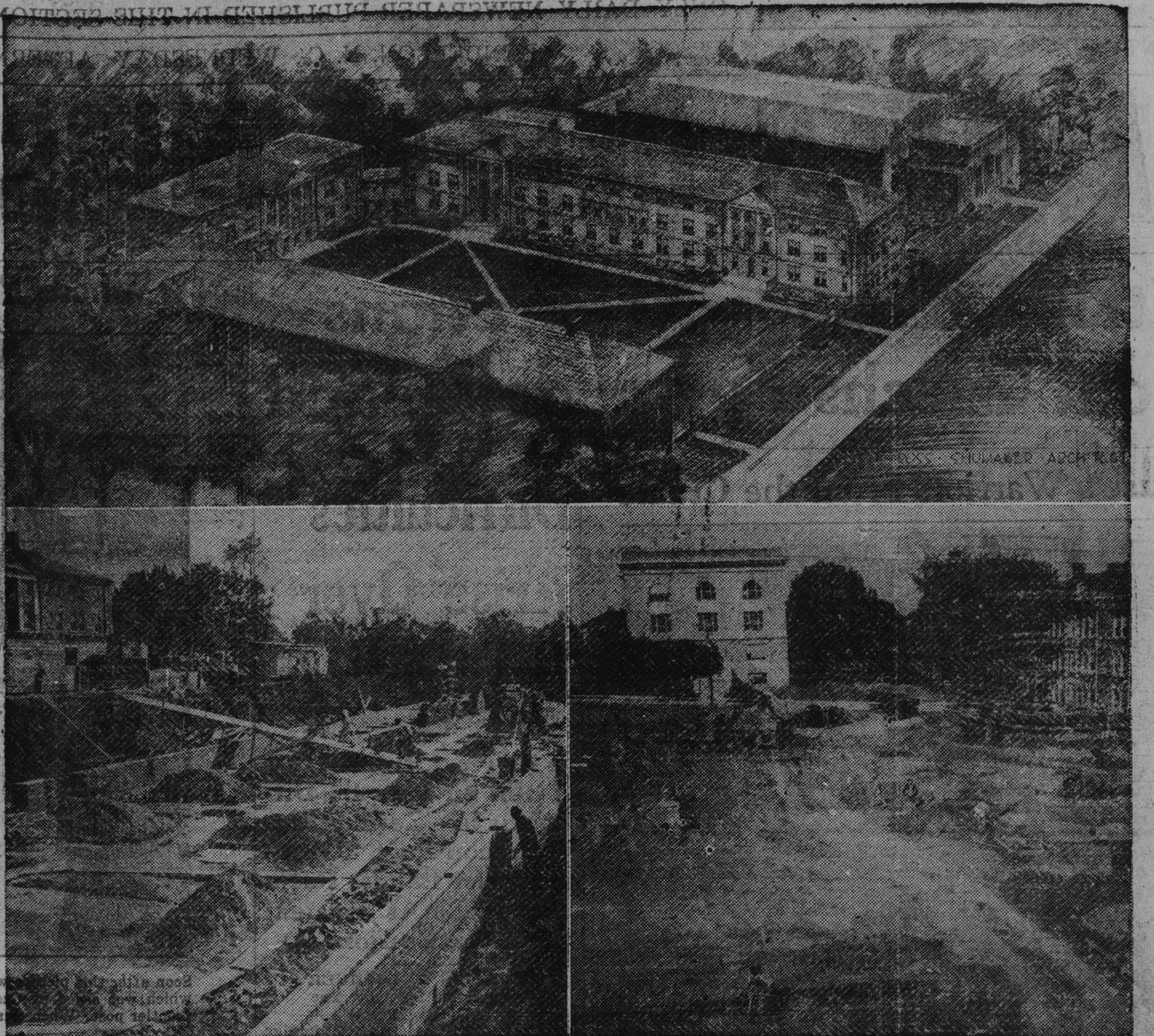
The four new dormitories which State College will have next year will house 710 more students.
