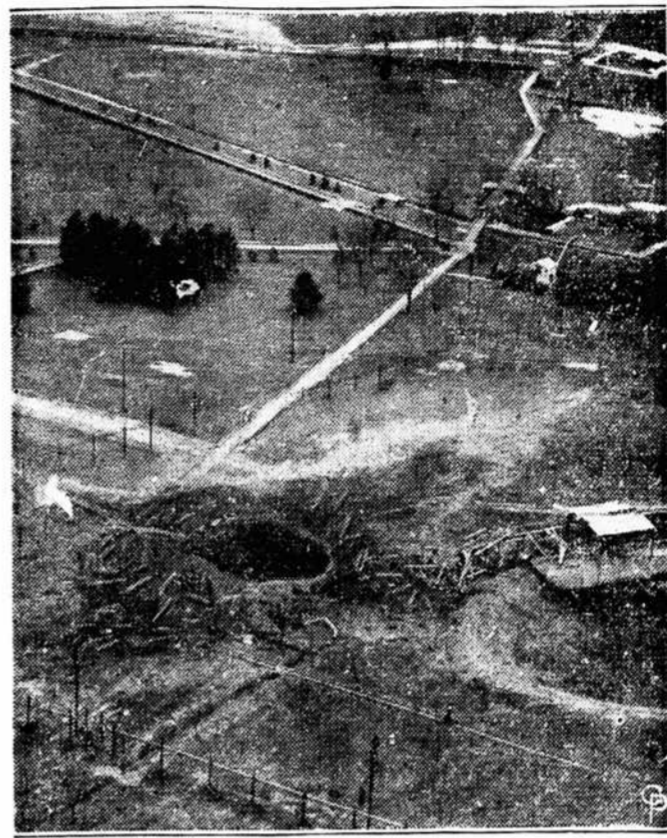
Terrific explosion of three tons of nitroglycerin near Gibbstown, N. J., at duPont plant, caused the death of two men, and left this 18-foot crater. The building was completely blown to bits by the detonation heard almost 50 miles away. Note how widely buildings are separated in interest of safety.
