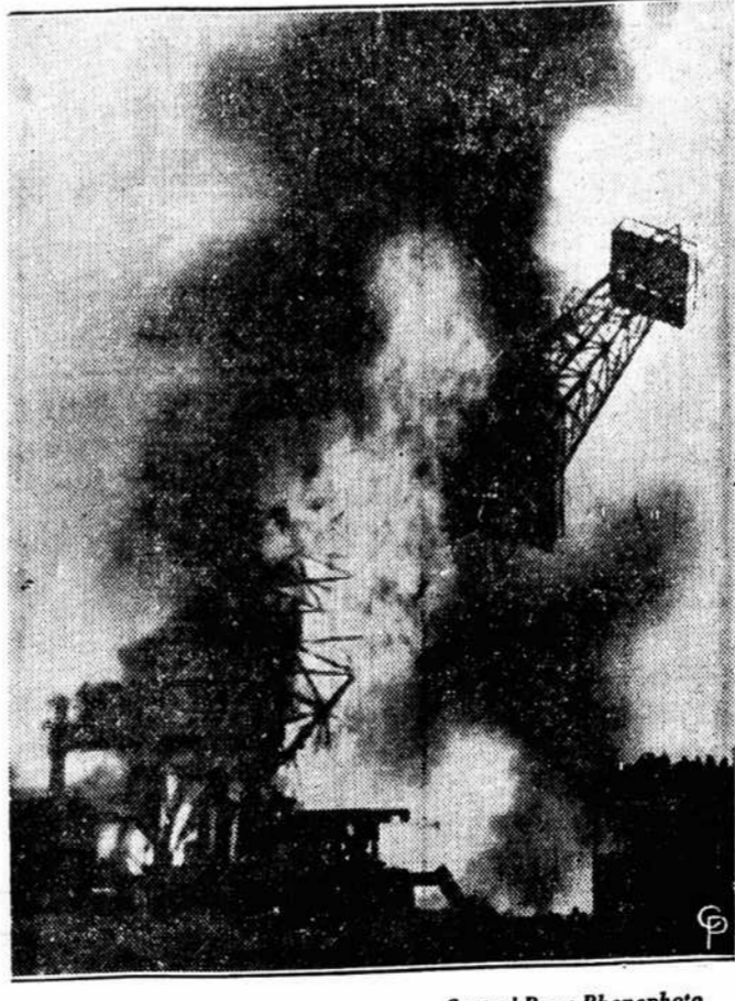
Static electricity, caused by seeping gas, ignited this oil well, belonging to the Ohio Oil Company, in El Segundo, Calif. A half-hour later the intense heat melted the base of the 125-foot tower, causing it to crash to the ground, as shown. Damage was estimated at $60,000, but nobody was hurt.
