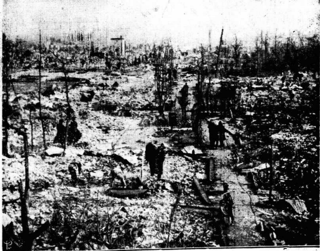
Here is what remains of the ravaged center of Shizuoka after the disastrous fire that burned 7,000 buildings to the ground in mid-January. The fire raged for 18 hours, leaving only a blackened waste in its wake. It was the largest fire suffered by Japan since the Hakodate holocaust in 1934, which destroyed more than 22,000 buildings and killed 2,165 persons.
