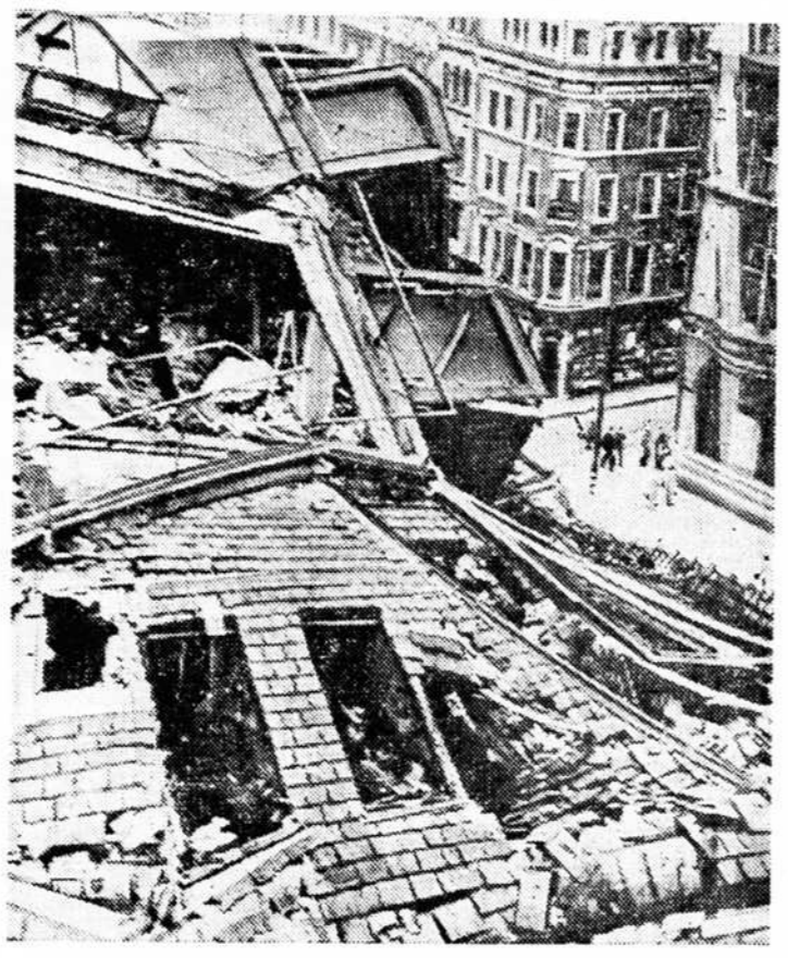
Shattered by Nazi bombs, this department store in London was thoroughly wrecked by the high explosives which German raiders dropped in the shopping district. Photo was cabled from London to New York.
