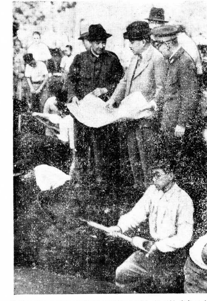
Engineering college students construct model air raid shelters in a crowded downtown district of Tokyo, according to the Japanese caption. Heavily populated Japan is extremely vulnerable to air attack.
