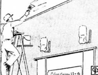
Sugar sacks hung over the lighting fixtures while a room is being redecorated keep the fixtures from being splattered.
