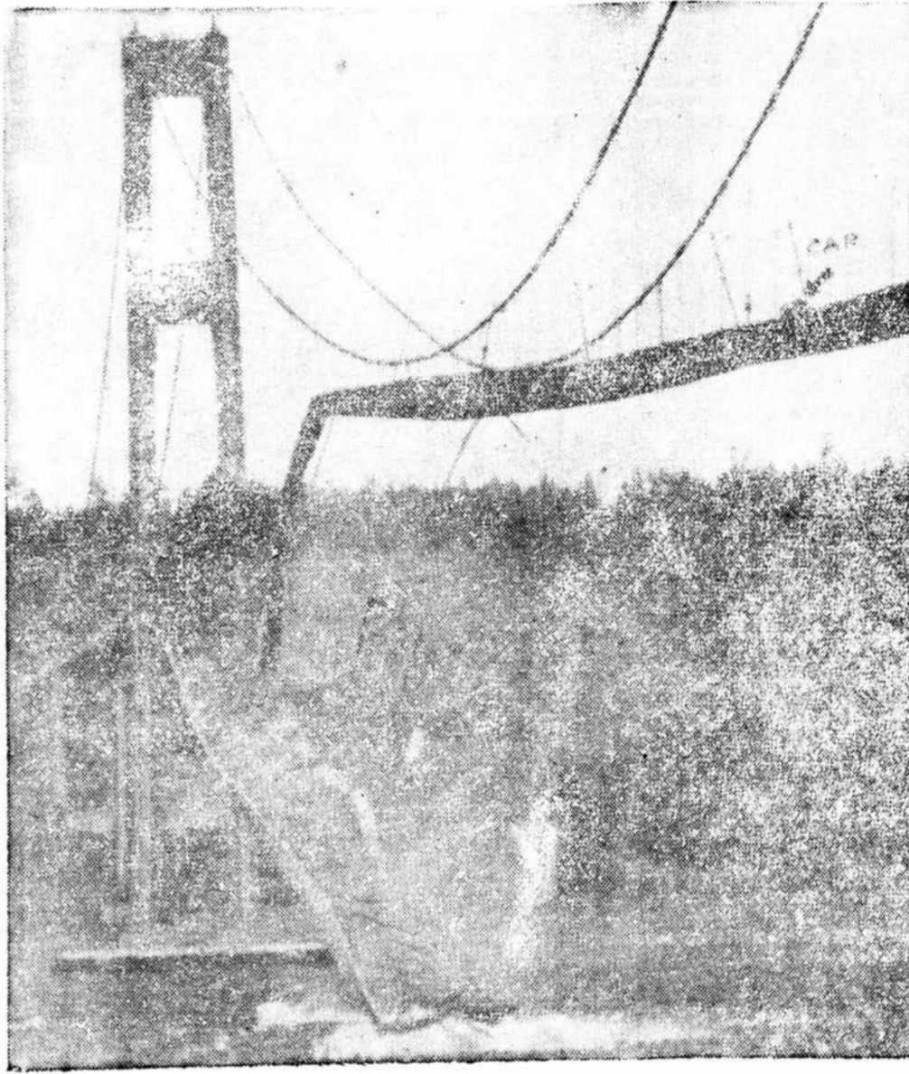
This photograph was snapped at the actual instant the central span of the new $6,400,000 steel and concrete Narrows Suspension Bridge, third longest span in the world, hit the waters of Puget Sound in Washington. The bridge crumpled under the impact of a gale and the central section fell more than 200 feet into the Sound. One motorist abandoned his car and crawled to safety just before the span collapsed. His car can be seen on the bridge.—Photograph by Bushford-Thompson.
