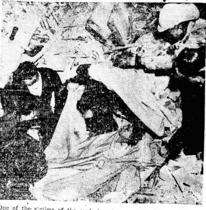
One of the victims of the explosion that demolished two tenement buildings in Cincinnati, Ohio, is removed from the wreckage. At least thirteen persons were killed. Investigators attribute cause of blast either to illuminating gas or to acids used by a chemist experimenting in the basement.
