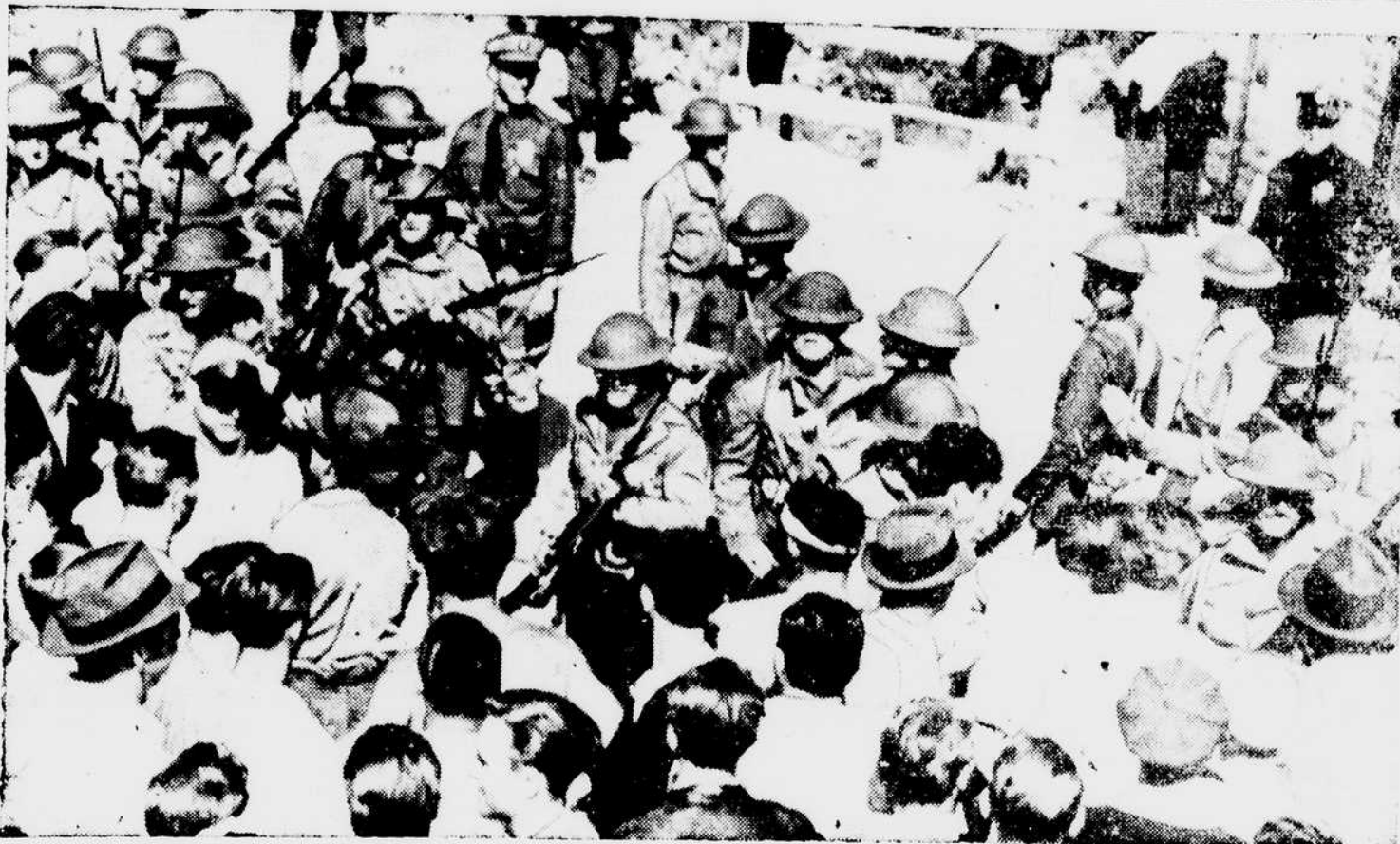
With fixed bayonets, steel-helmeted troops march on the North American Aviation plane plant in Inglewood, Cal., to seize the plant on direct orders from Washington. The people in foreground are mostly sight-seers who entered the troops. The pickets did not interfere with the soldiers.
