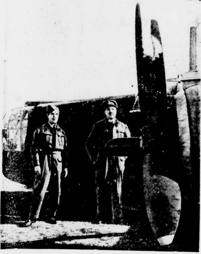
A Canadian R.A.F. squadron commander and his observer look over part of the plane that brought them home safely after being attacked by German fighter planes. The badly damaged plane could not rise over 20 feet, the tires were flat, the blade of the propeller was shot away, the turret was badly damaged and the navigator was winged in the arm. (Central Press)
