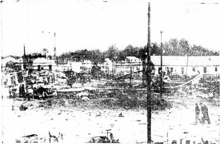
A SHATTERING EXPLOSION, followed by fire among the buildings of the Triumph Explosives Co., near Elkton, Md., caused the death of at least 13 workers. The toll of lives is expected to mount with investigation. This is a general view of the wreckage left by the blast. Benjamin F. Pepper, president of the company, said the Army, Navy and F.B.I. are directing the investigation. (International Soundphoto)
