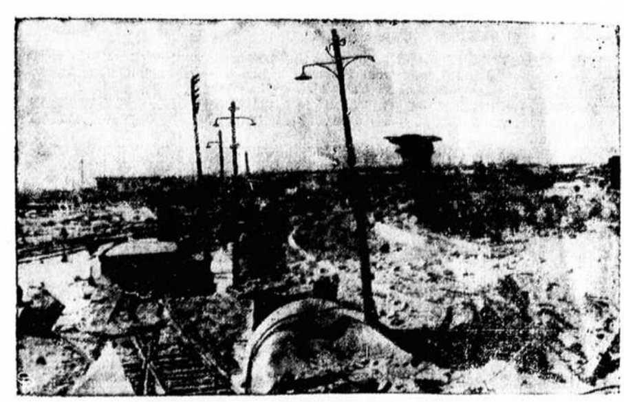
This is the ruin our fighters saw when they swept into the railroad yards at Messina, last stand of the enemy on Sicily. Rails he twisted, roadbeds are torn and rolling stock has vanished under the day-long storms of our bombings. (International Soundphoto.)
