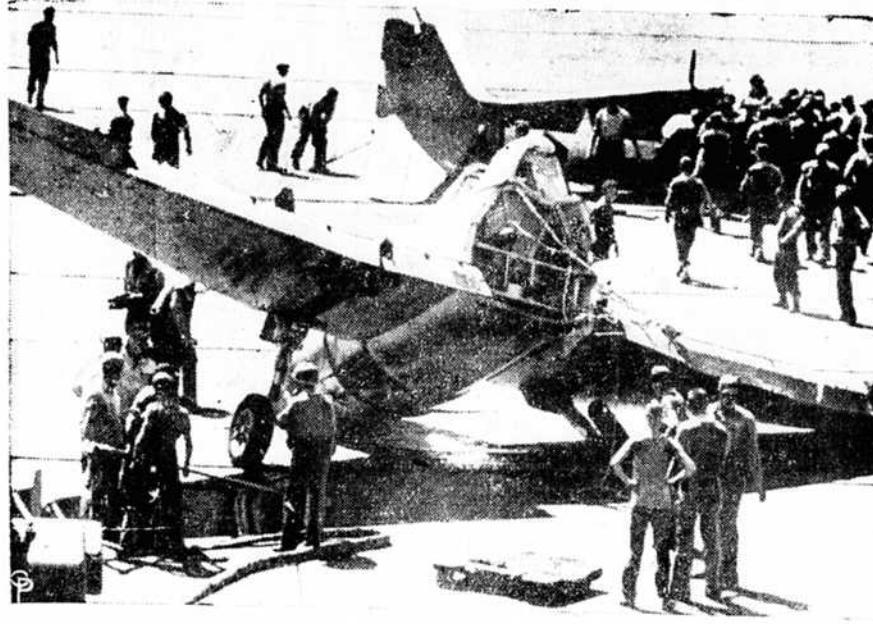
THE CRASH CREW aboard a U. S. carrier clears away the wreckage of a plane that had crashed in two on the flight deck. The craft, piloted by Lt. Charles L. Mountenot, Edgewater, N. J., was hit by fire while attacking Tarawa and the hydraulic system was shattered. As it was set down on the carrier deck on one wheel the landing hook caught and the plane tore into two sections. (International)
