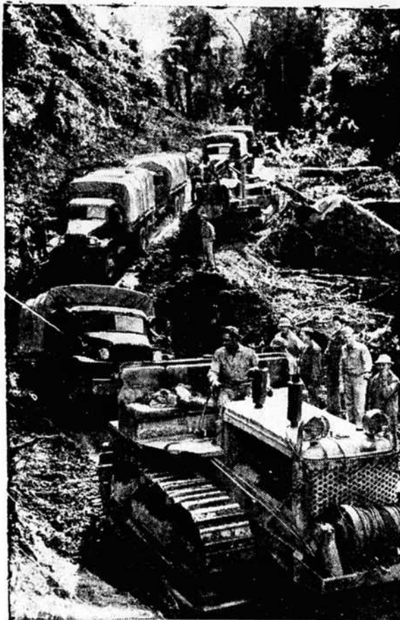
A CATERPILLAR comes to the rescue of a truck caravan on the Ledo supply road to China which has been hacked through the jungles and mountains by American engineers. The lead car had been bogged down in the roadway which had been softened by a rainfall. (International)
