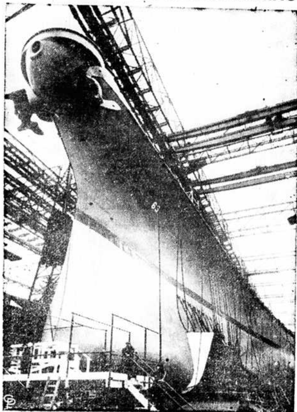
Called by the Navy the "world's mightiest," the U. S. S. Missouri, 15,000-ton battleship, is shown on the ways at the Brooklyn Navy Yard. The new dreadnaught, which will be launched Saturday, is 800 feet long, 119 feet less than the Normandie, U. S. Navy photo (International)
