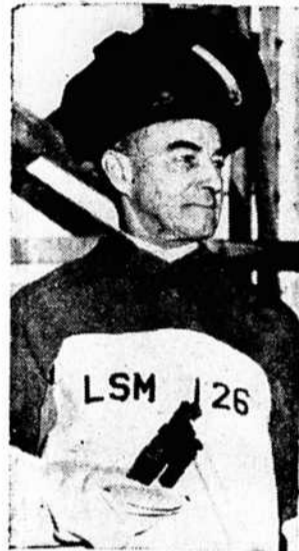
WEARING a welder's outfit, Adm. Thomas C. Hart is shown as he officiated at the laying of two keels for mechanized landing ships to be constructed at the Charleston, S. C., Navy Yard. This is an official U. S. Navy photo. (International)
