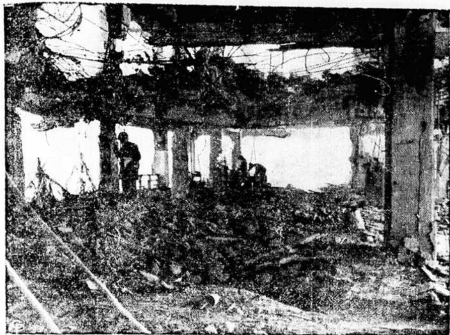
The wrecked Jap steel and concrete blockhouse on N mar island, on Kwalein atoll, is mute but striking testimony to the ferocity of the land, sea and air bombardments that softened up this section of the Marshall Islands for our invasion forces. This effective barrage is credited to the small price in lives we paid for capturing that strategic mid-Pacific bastion. (International Soundphoto)
