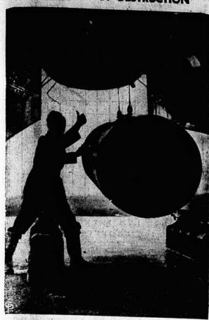
ON WIRES that only seem dangerously thin, a 4,000-lb, bomb is holsted very carefully into its rack aboard a giant Lancaster about to fly from Liviland on a dission to Germany. The armorers' "thumbs up" shows that all goes well with the delicate job.
