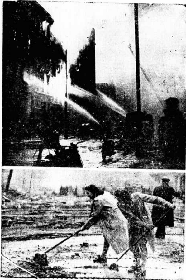
High pressure streams of water are turned on one of the buildings set afire (top) during a recent raid on London by Nazi bombers. The fires were quickly brought under control and the following morning many residents of the city helped to clear rubble from the streets. Two young girl volunteers are shown (bottom) aiding the clean-up. (International)
