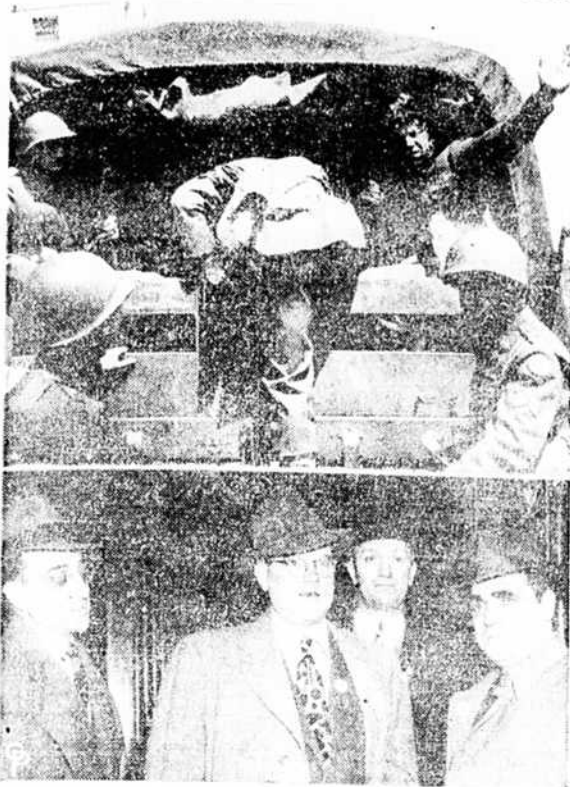
ARMY TROOPS leave the Montgomery Ward plant (top) after Henderson victory of Commerce Wayne C. Taylor, in charge of the Government, said "there is more to be done for their recovery." Also shown in front of the plant (bottom) and the company are held if the N. I. F. B. so decided. L. to r.: Henry D. Hoffmann, Leonard Levy and Samuel Wolfshok.
