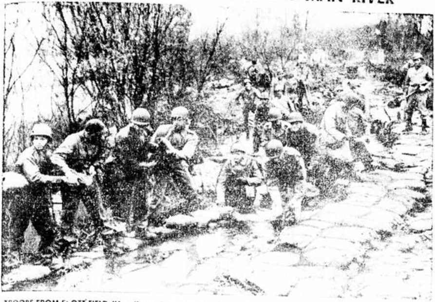
TROOPS FROM SLOTT FIELD, ILL., pile sandbags against the crumbling banks of the Mississippi River at nearby Hajo in an endeavor to save the town from the rain-swollen river, now at its highest level in 100 years. The total acreage flooded by "Old Man River," the Illinois and Missouri is estimated at 1,212,000. Forecasts of more rain have prompted calls for more men to raise the levees. (International Sunshoto)
