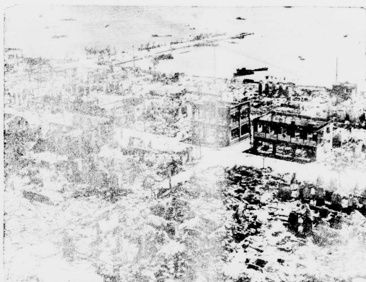
JUST THE WALLS of buildings remain after U. S. land, sea, and air forces had shelled and bombed Gapan, capital of Saipan, in the Marianas. When this photo was taken, the city was still the scene of bitter street fighting between our forces and the retreating Japs. Since the island was invaded, our troops have killed approximately 10,000 Japanese soldiers and retained many.
