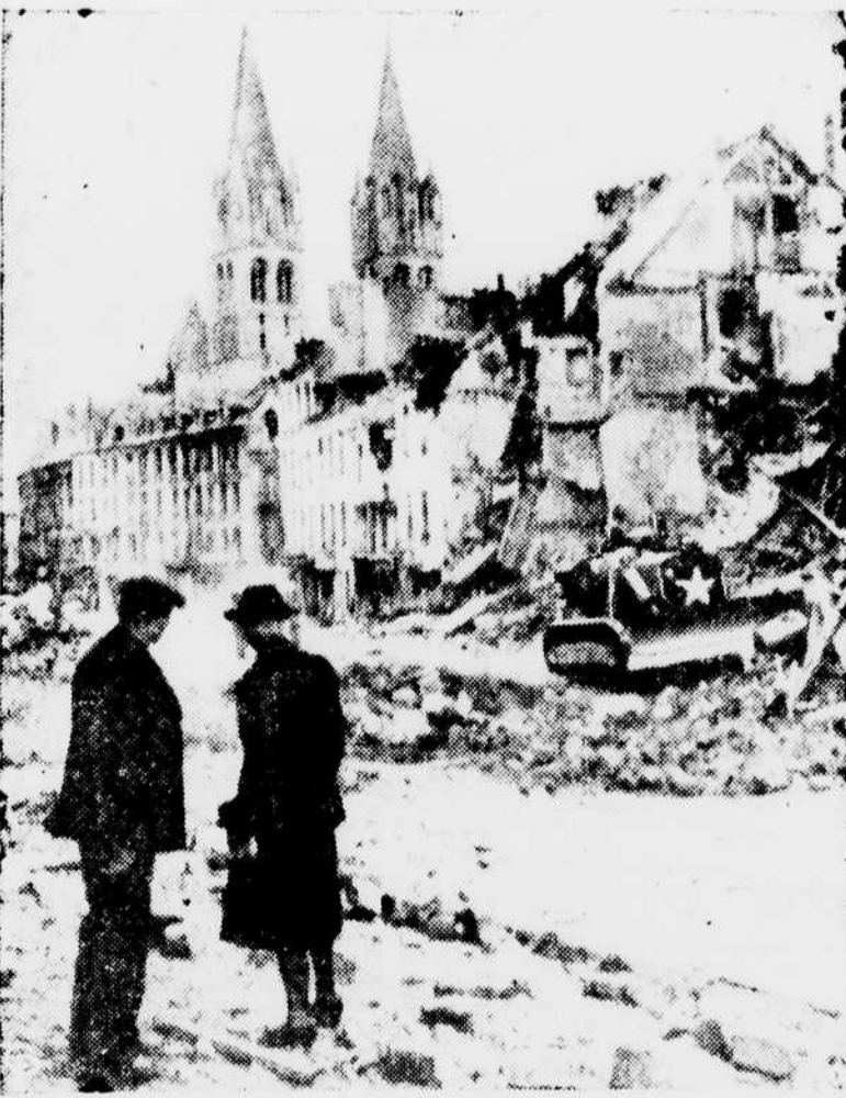
TWO FRENCH CIVILIANS gaze at the spires of Abbeys Aux Hommes, in Caen, France, which miraculously survived the heavy bombardment of the city which preceded its capture by the Allies. A bulldozer (right) is already clearing the debris. Signal Corps Radiophoto. (International)
