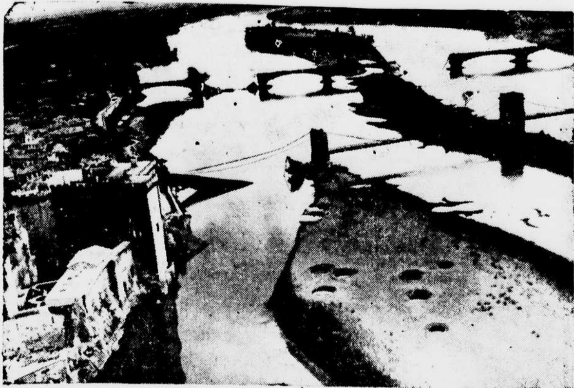
HERE IS ONE OF THE REASONS why the German forces couldn't retreat in southern France. Bridges spanning the famous Rhone River at Taronnes were made useless by Allied bombers to hinder the flight of Nazi troops and supplies. Pock marks on one of the islets (right foreground) indicate some near hits. (International)
