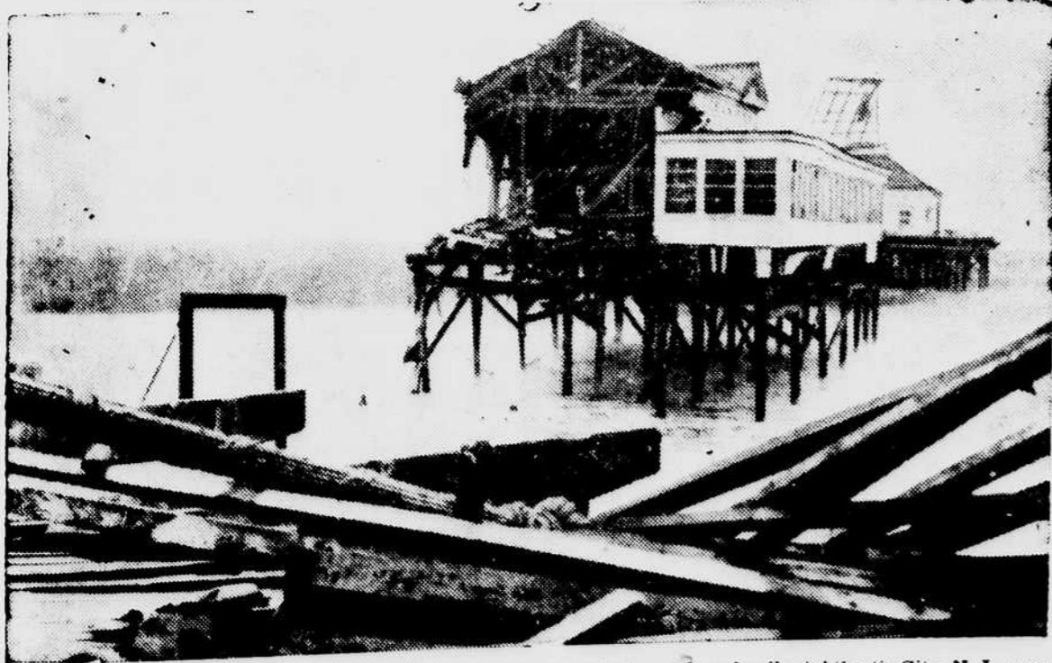
THIS VIEW OF THE WRECKED Heinz Ocean Pier and part of the shattered boardwalk at Atlantic City, N. J., was taken after the hurricane had struck the summer resort and furiously destroyed property and utilities. All along the eastern seaboard, the gale is said to have caused damage estimated at $30,000,000. (International)
