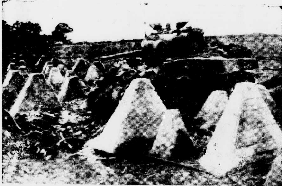
AMONG THE WIDELY ADVERTISED features of Germany's Siegfried line have been the steel and concrete tank obstacles in the Aachen area. These have become known as "Dragon's Teeth," but above is demonstrated how these "teeth" are being pulled. U. S. Engineers have been blasting many paths and through one of these passes a 1st Army tank hammering its way into Germany. Signal Corps photo. (International)
