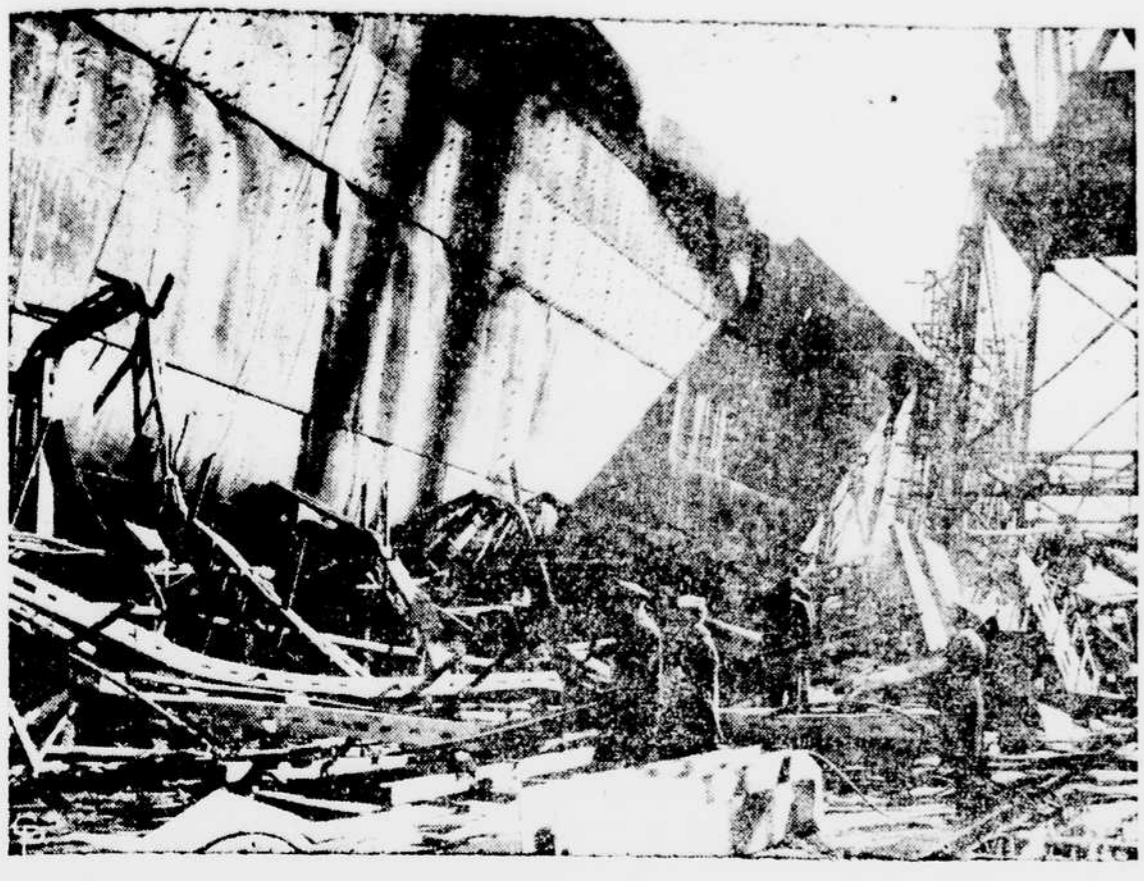
Here is a view of the damaged construction ways containing a partially built cargo ship in the Kearny, N. J., yard of the Federal Shipyards and Drydock Company, after it was swept by flames burning 200 feet high. The fire of undetermined origin was being fought by fire companies from Kearny, Jersey City and Newark, as well as three Coast Guard fire boats. (International)
