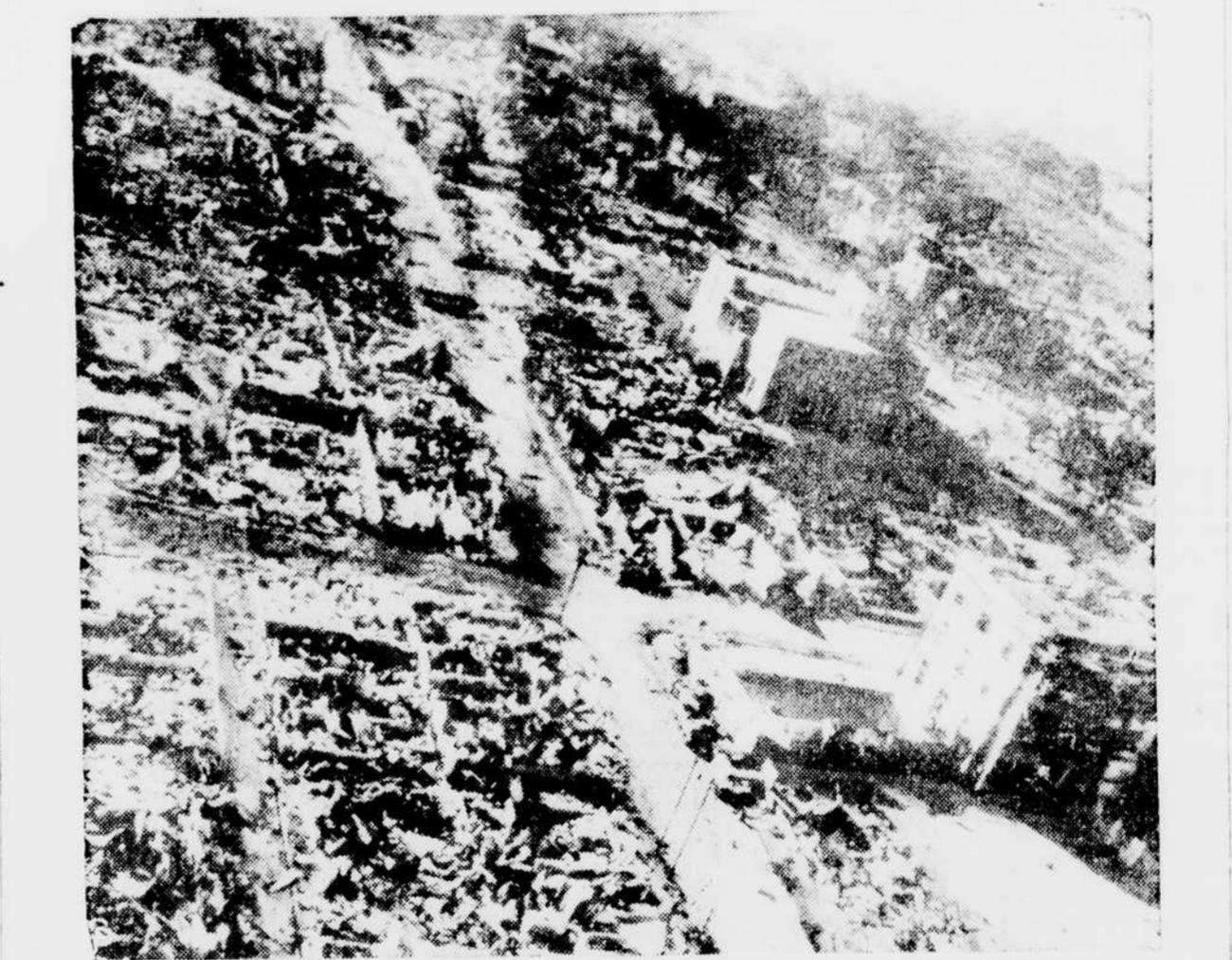
HERE IS AN AIRVIEW of a war-shattered section of the residential district of Manila after the Japs had burned it in their retreat from the Philippine capital. At right center can be seen a wing and the swimming pool of the Philippine Women's University, at upper right the Masonic Temple. Signal Corps photo. (International)
