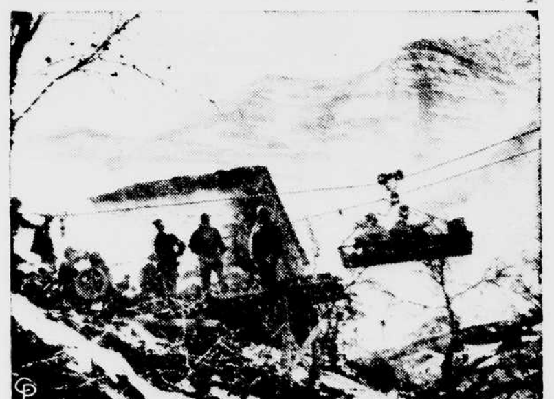
CONSTRUCTED BY U. S. ENGINEERS in nine hours, this tramway is shown beginning its 1,600-foot journey up Mt. Serrasciccia, Italy, for Fifth Army casualties. The trip by litter bearers over the mountainous terrain formerly took six hours, but by tramway the wounded can be evacuated in four minutes. OWI Radiophoto.
