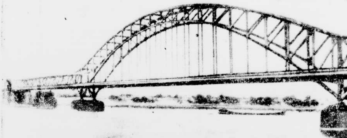
EXACTLY AS IT APPEARS in this peacetime picture, the bridge across the Rhine at Remagen was found undamaged and ready when the U. S. First Army struck suddenly and seized it for putting armor and infantry across into the heart of Germany—the first war-time crossing of the Rhine since Napoleon's day. First Army spearheads are reported still advancing miles beyond the bridge. (International Soundphoto)
