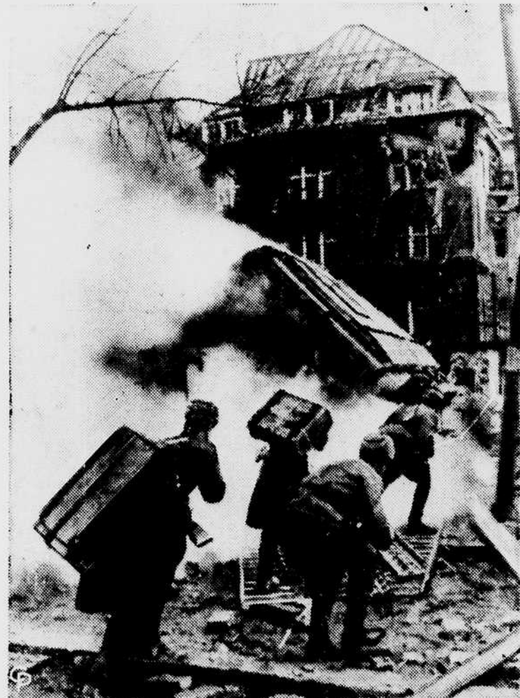
A GROUP OF RED ARMY SAPPERS advances toward a building in Breslau, Germany, intent on blowing it up. They carry loads of explosives, and a bullet fired into their dangerous burden would blow them up. The Russians succeeded in blasting the building, which had been converted into a stronghold by the Nazis. (International Radiophoto)
