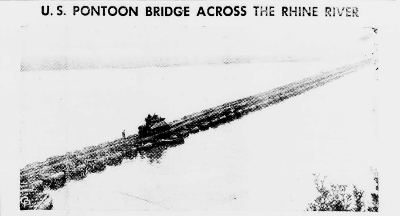
U. S. PONTON BRIDGE ACROSS THE RHINE RIVER ONE OF A NUMBER of pontoon bridges spanning the Rhine is pictured shortly after U. S. Army engineers had constructed it to replace the railroad bridge that had collapsed at Remagen. Large numbers of men and huge amounts of equipment are reported to be pouring across these structures as the all-out Allied drive gains momentum. This is an official U. S. Signal Corps photo.
