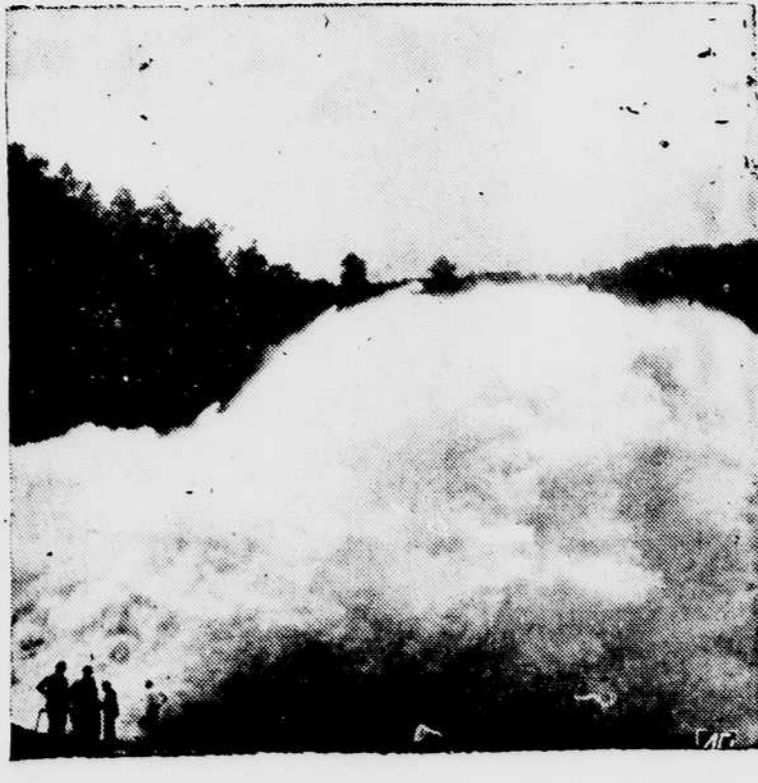
Right: a close-up of the roaring torrents. The water is traveling at a velocity of about 150 feet per second and is deflected more than 100 feet and air and spray fan-shaped as spray about 400 feet down stream to reduce erosion of the river bed. (Ap Photos.)
