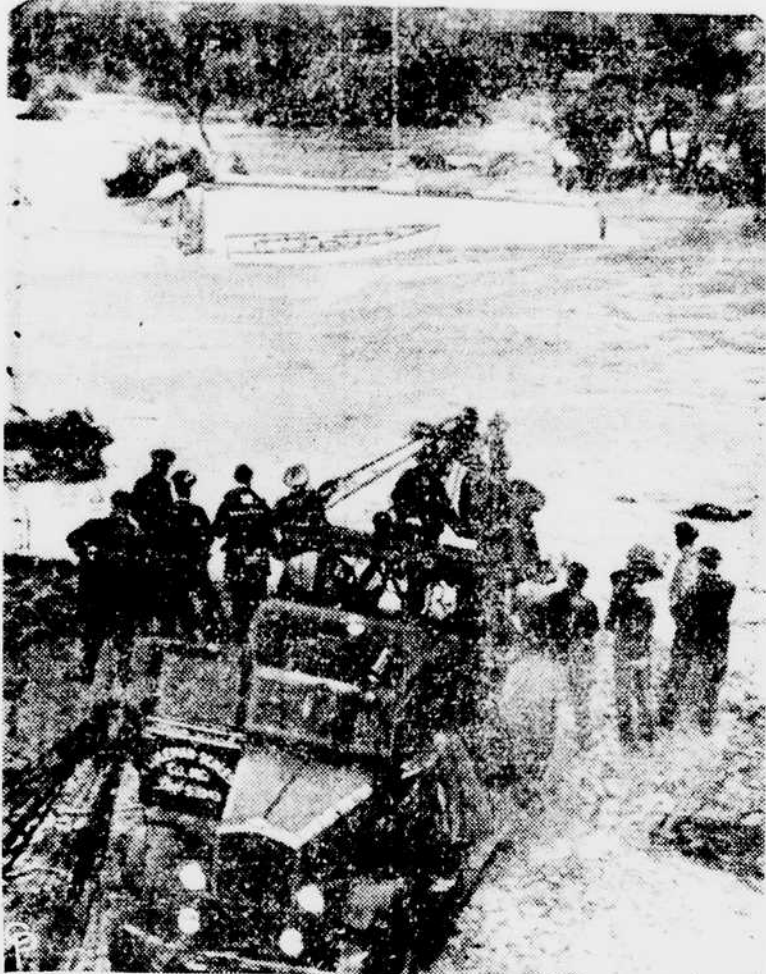
WRECKER CREWMEN recover from Gillies Creek, near Richmond, Va., the inter-city bus which, breaking through a bridge, carried two passengers to death and 43 others to danger in the rain-swollen flood. The two who died were Donna Jean Hammett, an infant, of Delta, Pa., and Pte. Julius Slobin of Brooklyn, N. Y. (International Soundphoto)
