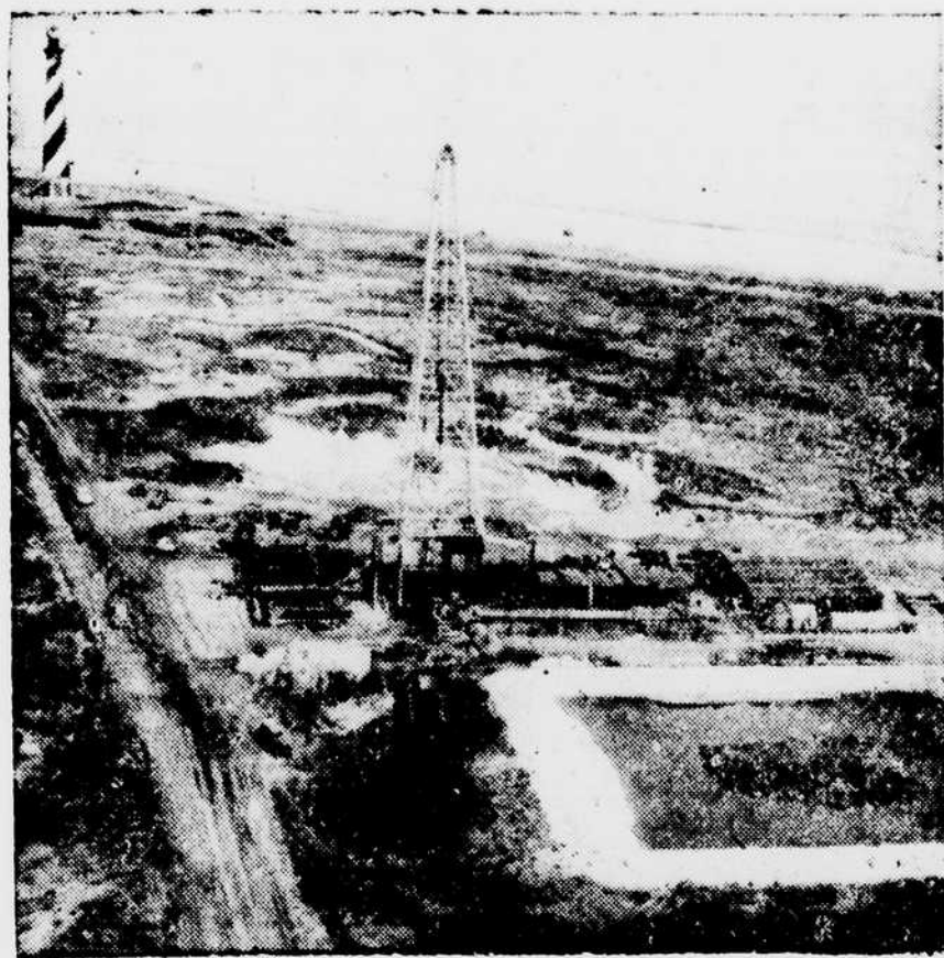
Near the historic 197-foot lighthouse (background) at Cape Hatteras, N. C., rises the 168-foot rig (foreground) of Esso No. 1 well where drillers of the Standard Oil Company of New Jersey have bored more than 3,000 feet in quest of oil on the coast. The square pool (right foreground) is a storage basin for drilling mud. The drilling is expected to continue to a depth of 8,500 feet. (AP Photo.)
