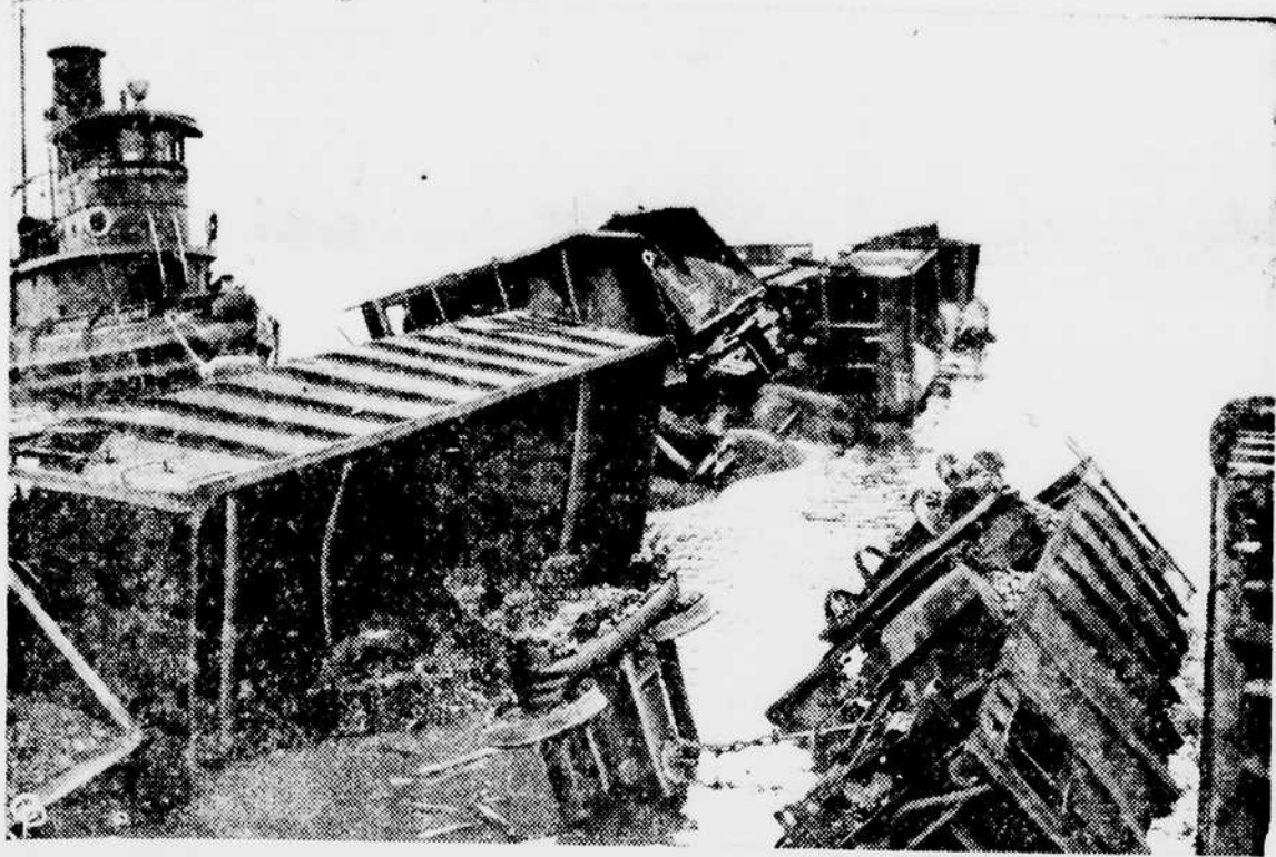
TONS OF PRECIOUS COAL are spilled into the Hudson River, off Weehawken, N. J., just when the miners' strike has made the need for the fuel so acute. The coal was lost when a railroad car float sprang a leak and toppled eight of sixteen railcars into the river. Clearance and salvage would take two weeks, according to railroad men who investigated the odd river-crossing freight train accident. (International)
