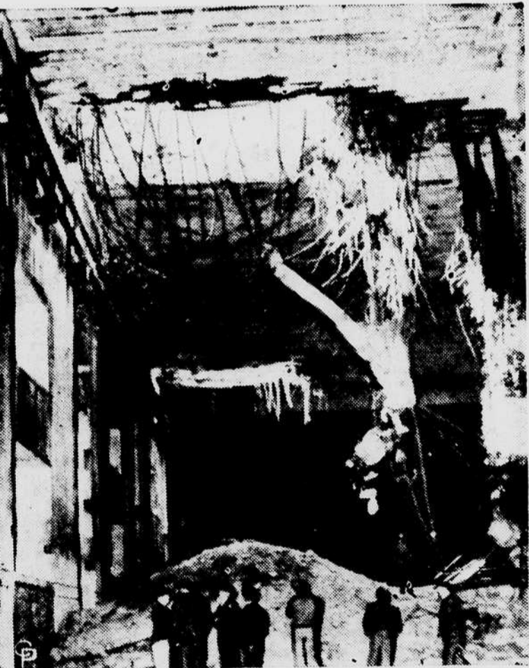
AMERICAN AND BRITISH OFFICERS study two huge holes ripped in the roof of one of the submarine pens at Farge, Germany, by heavy bombs dropped in experiments conducted by the U.S.A.A.F. and the R.A.F. Only two of the big missiles have succeeded in breaking through the steel and concrete walls which are 14-feet thick. (International)
