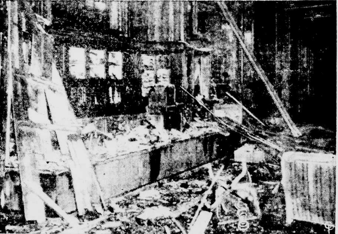
LITTERED WITH DEBRIS, the fire gutted lobby of the LaSalle Hotel in Chicago, Ill., bears mute testimony to the fury of the flames that swept through the hotel in the early morning hours killing 51 and injuring over 200 persons. The fire is believed to have started in the coffee shop of the hotel. (International Soundphoto)
