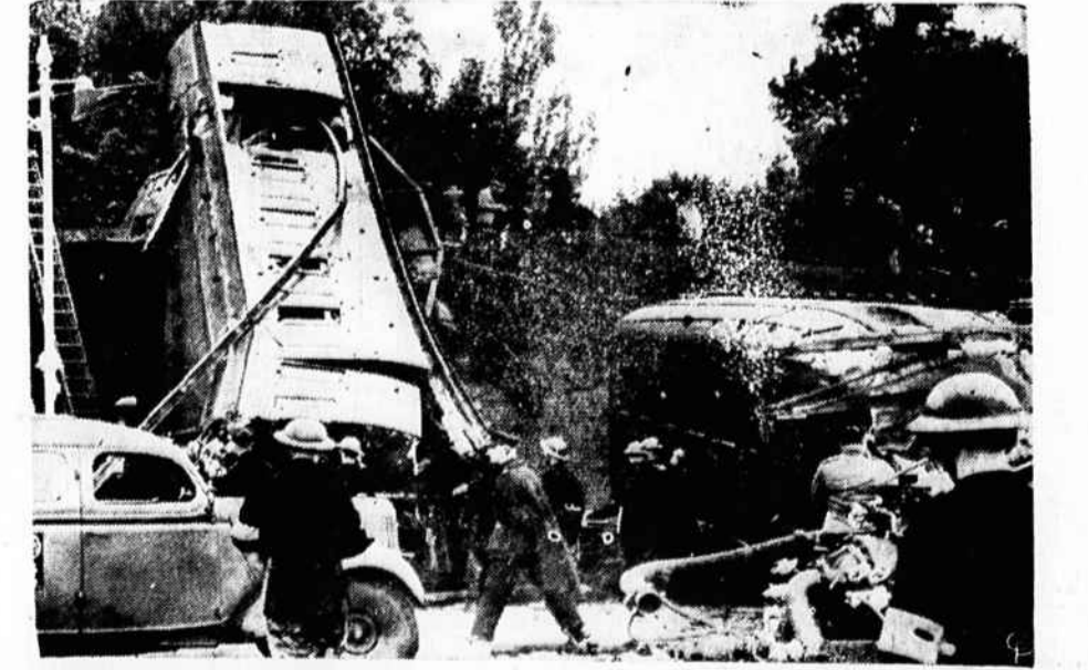
POLICE AND FIREMEN comb the wreckage for survivors of a passenger train that plunged down the embankment at Catford, England, after heavy rains which are believed to have undermined the tracks. One man was killed and twenty injured. Heavy damage was caused by the violent gales and floods. (International)
