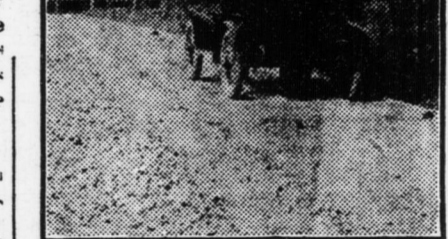
A POORLY CONSTRUCTED MACADAM ROAD.
