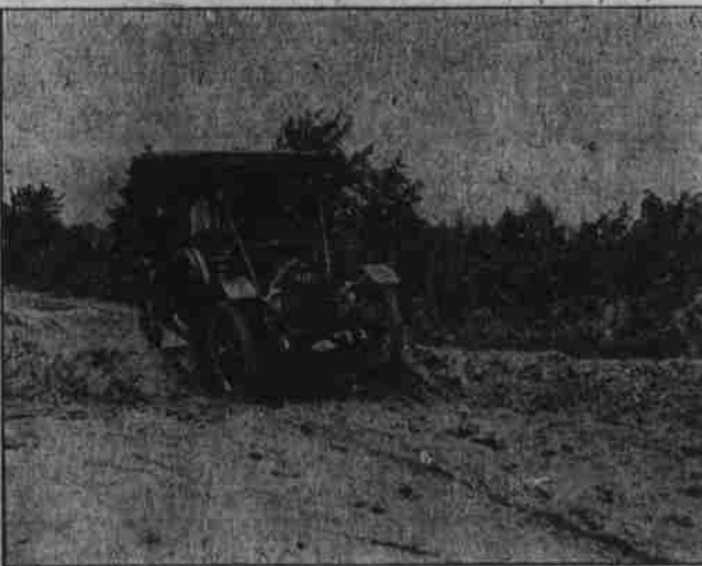
Fig. 2. Road with steep grade (average 10 per cent.) Travel made more difficult by uneven surface of road; large stones project above the road.
