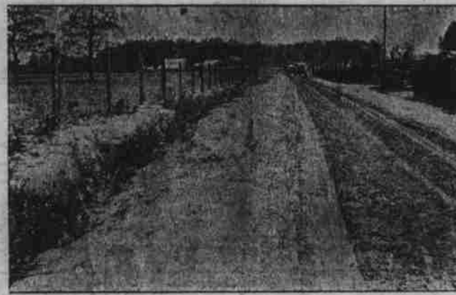
Fig. 6. The old way of throwing dirt from ditches on one side of road preventing drainage from road into ditch. The scene is in Craven County.
