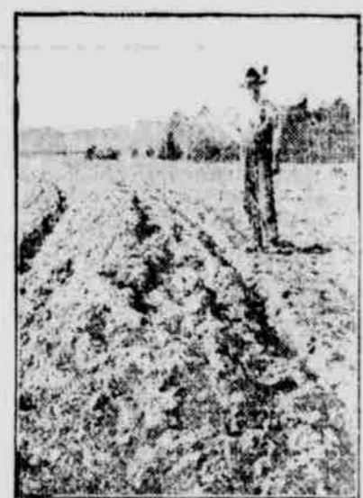
The First Step in Building a Terrace is to Back Furrow a Strip About Four Furrows Wide.
